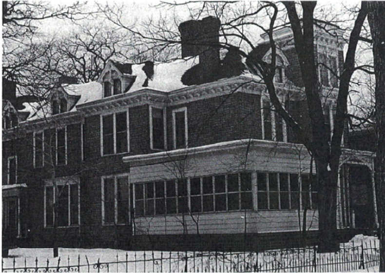
The Sanborn house, still standing at 143 Virginia Avenue in St. Paul.
